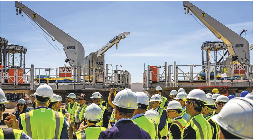
The Revolution Wind construction hub at the Port of Providence in Providence, Rhode Island.
