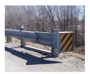
52. Upon head-on impact, the guardrail extruder terminal is designed to move rearward along the guardrail, shearing or bending the posts and extruding the W-beam guardrail into a flattened ribbon, while bending the guardrail away from the colliding vehicle and traffic. This process is intended to absorb the kinetic energy of the impact while bringing the vehicle to a controlled stop, and to avoid the spearing and rollover risks associated with prior end terminal designs.
